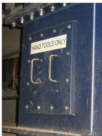
Figure 3 – Dust duct access door
