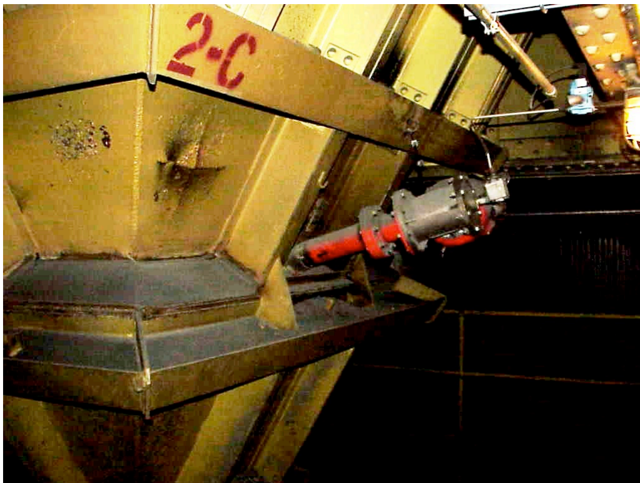
Figure 6: Air cannon installed on transition hopper.
