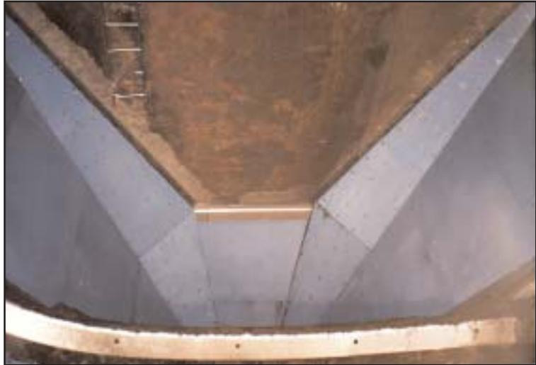
**Figure 10.** TIVAR® 88 liner installed on clean out plates and gunite sloping wall surfaces
