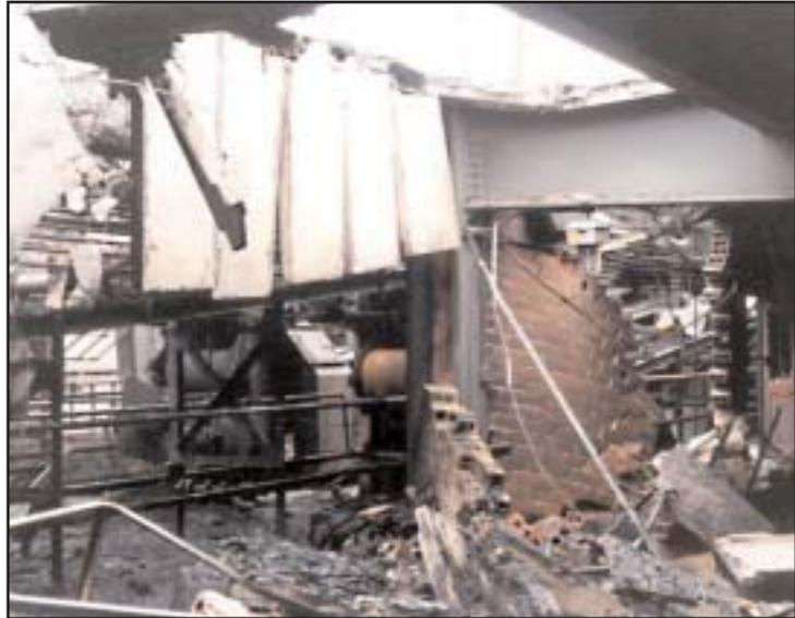
**Figure 2.** Looking from the boiler room into the conveyor room at 5B bunker drop chute. The three people injured were at this point when the conveyor room “lit-up”.
