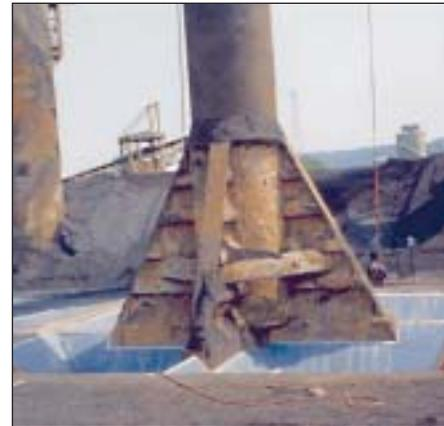
**Figure 8a. Kammer reclaim hopper - during TIVAR® 88 installation**
