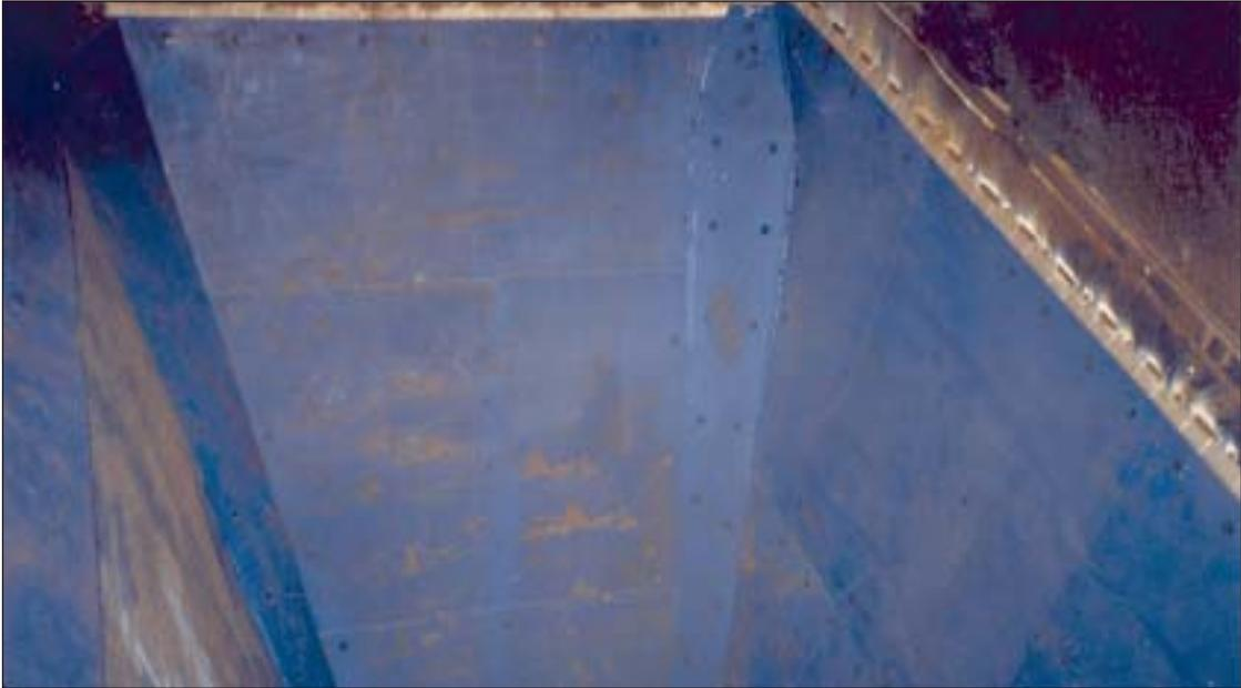
**Figure 7. Typical hopper liner installation in progress**
